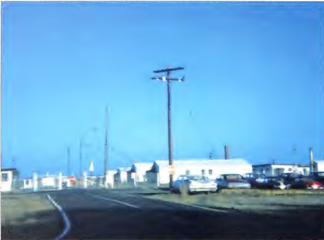
Figure 4.20. View from Hartshorne Drive looking east at Ready Barracks, NIKE launch site, circa 1958. A parking lot and several parked cars are seen west of the Hartshorne Drive's northbound lanes. An approximate 50-foot by 180-foot asphalt parking area is presently extant in this location (GATE 20157).
